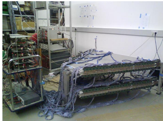
Figure 5: Structure of each sector and setup during the commissioning.
